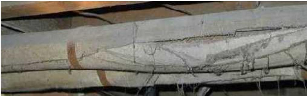
The above photo shows a typical asbestos insulated heating pipe found in older homes.
